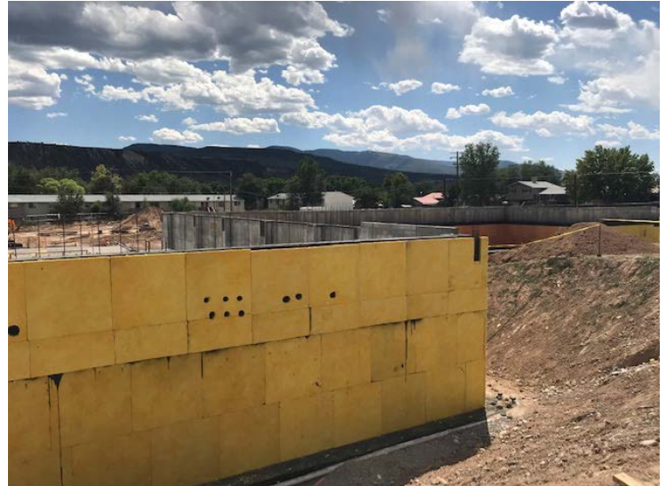
AREA A RETAINAGE WALLS ARE COMPLETE WITH WATERPROOFING AND INSULATION COMPLETE
