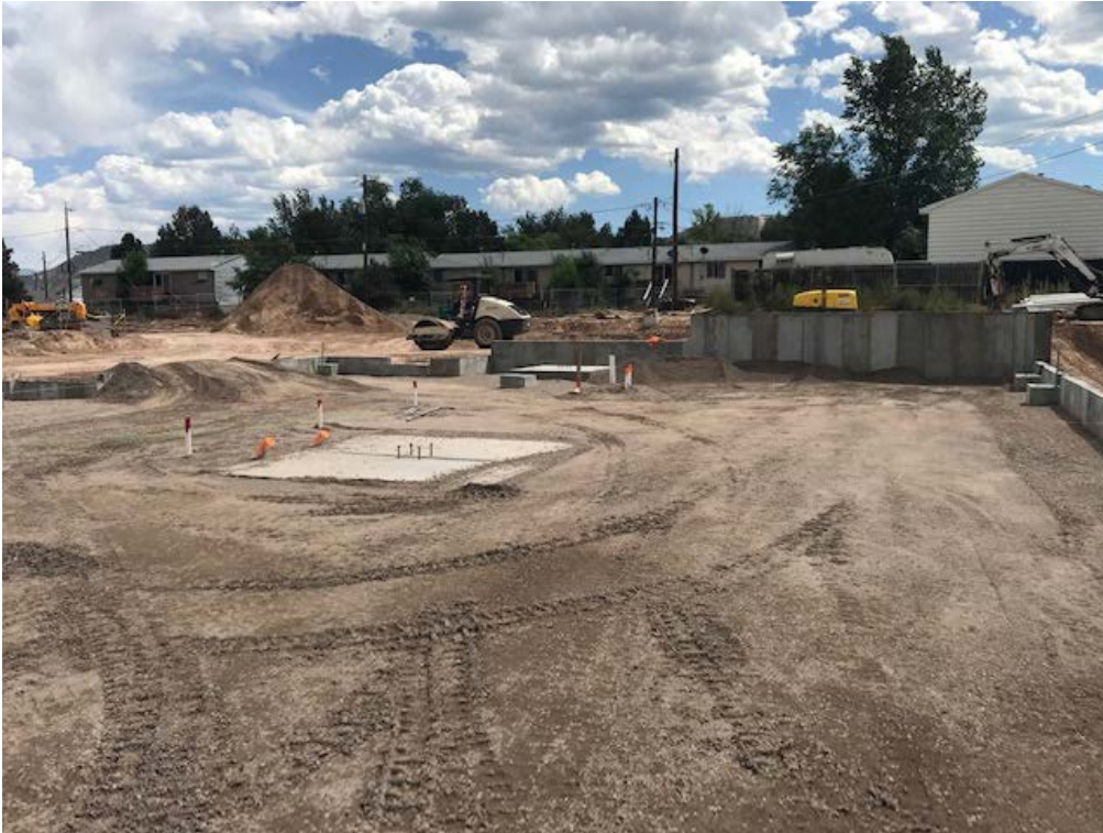
AREA D UNDERGROUND UTILITIES AND SLAB ON GRADE PREP
