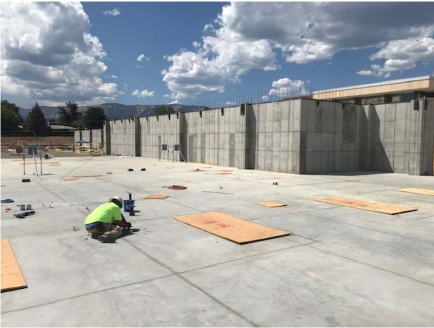
AREA C SLAB ON GRADE
