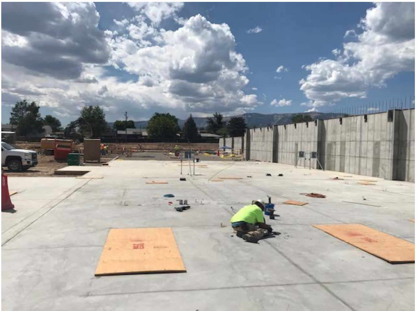
AREA C SLAB ON GRADE
